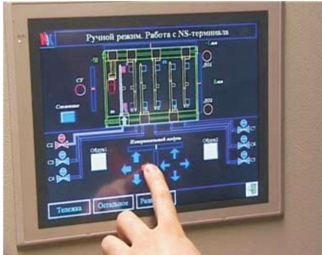
Fig.19. Automatic system control panel EMATEST-PIPE.
