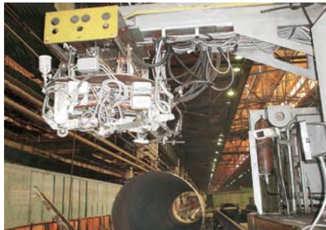
Fig.10. EMATEST-PIPE for spiral pipes inspection - Volzhsky Pipe Plant, Volzhsky (Russia).
